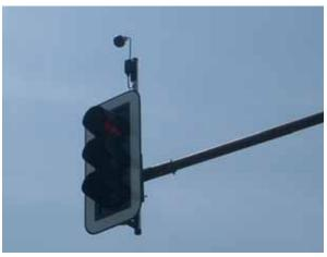
This above-ground sensor allows quick and flexible installation.
